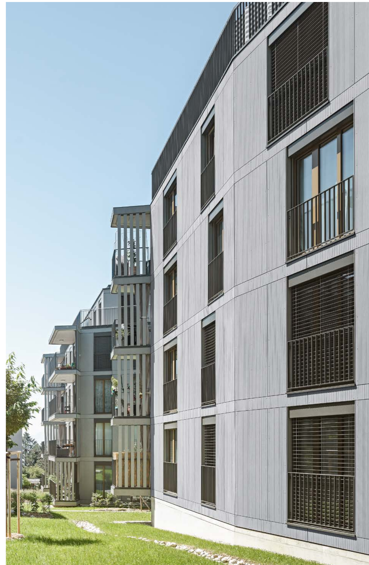
Fiches Nord, Lausanne, Switzerland. Architect: Züst Gübeli Gambetti Architektur und Städtebau AG, Zurich, Switzerland. Photographer: Roger Frei, Zurich, Switzerland.
