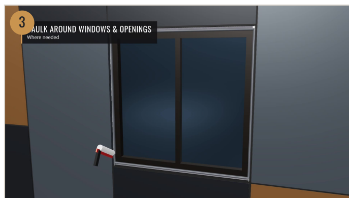
Caulk around windows and openings where needed.
