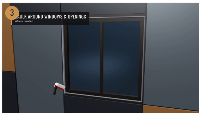
Caulk around windows and openings where needed.
